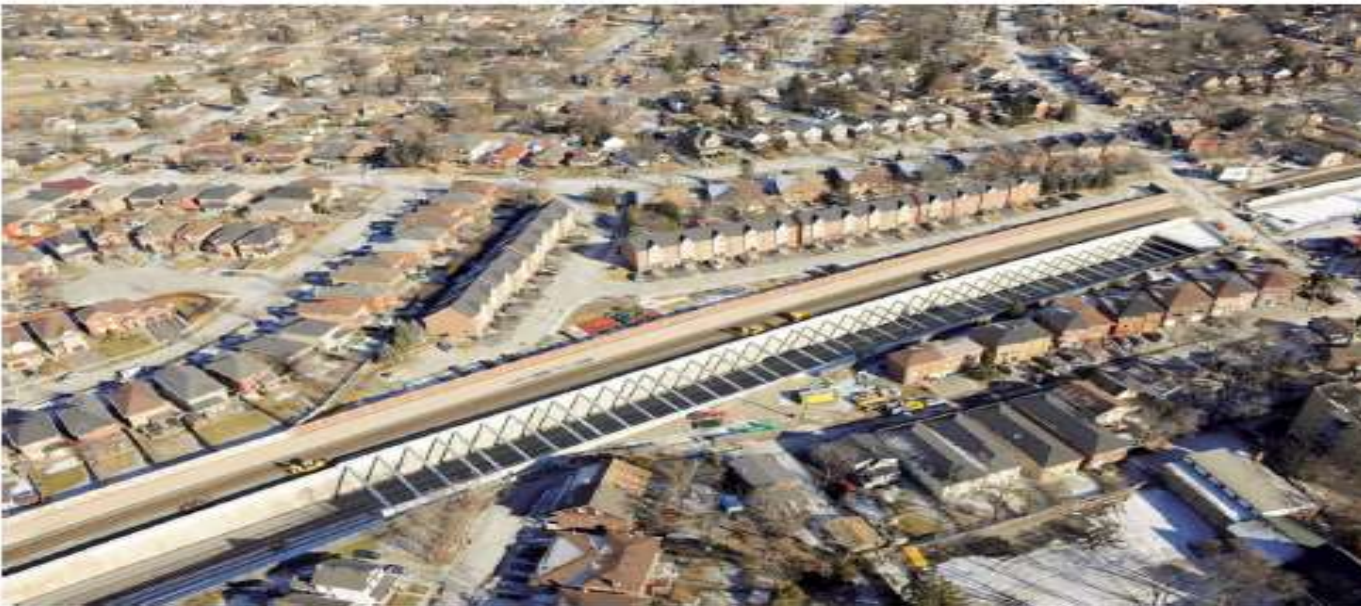
Weston Tunnel – January 2015
